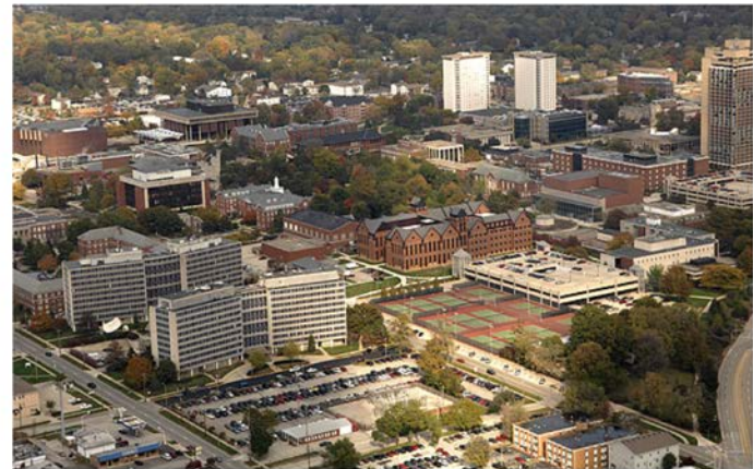
Aerial view of Illinois State University looking northeast.
