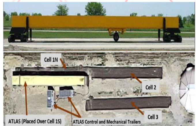
Google Satellite View of the Construction Site Showing Overall the Constructed Test Cells (top image), ATLAS accelerated pavement testing (bottom image)
